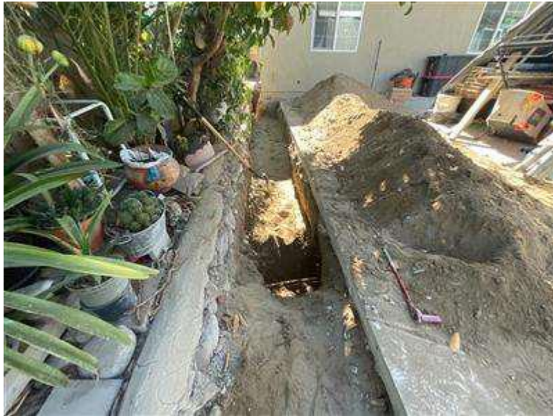
Photo 1 provided by Southern California Gas Company depicts the backyard jobsite. (Exh. 1.)
