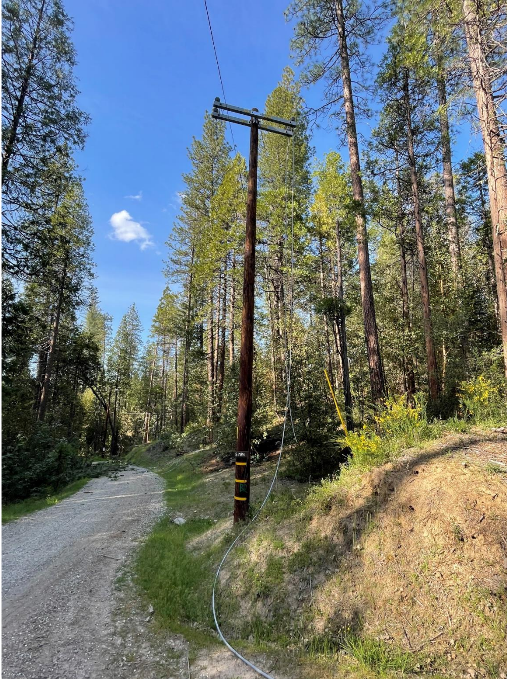
Figure 8 Photo taken by responding troubleman showing wire down.
