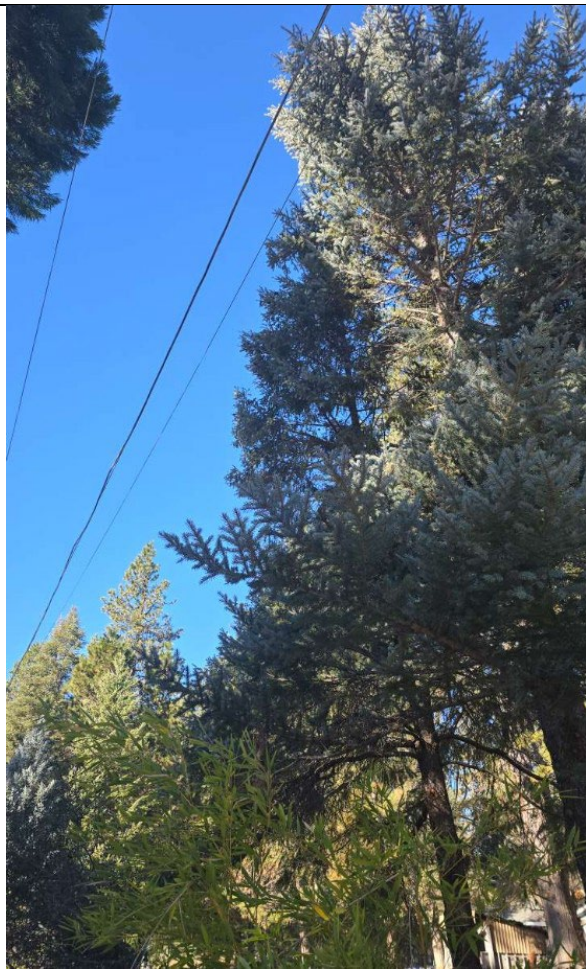
Photo 3: Douglas fir branch 7.7 feet from distribution conductor. Photo taken facing northeast from the pole.
