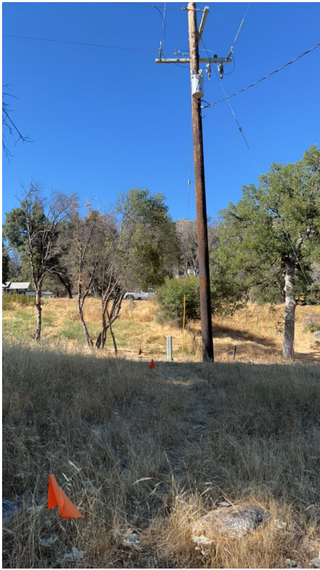
Item3IA1Img2: Overall north view
