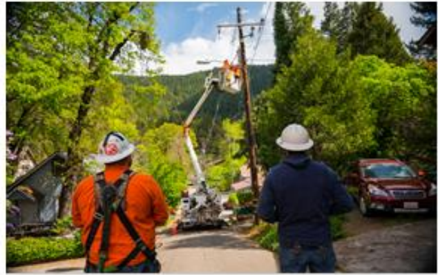
Figure 8-13: Line Crews at Work
