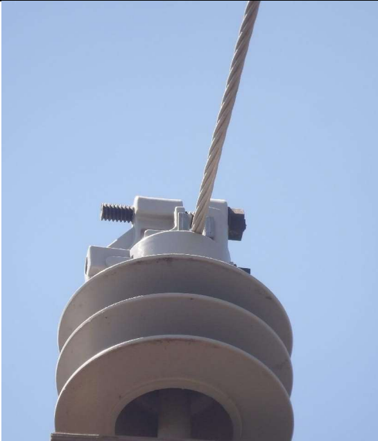
Item1IA1Img1: No Covered Conductor Present
