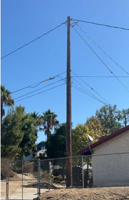
Item1IA1Img1: No covered conductor present
