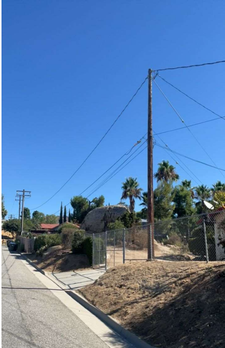
Item1IA1Img2: No covered conductor present
