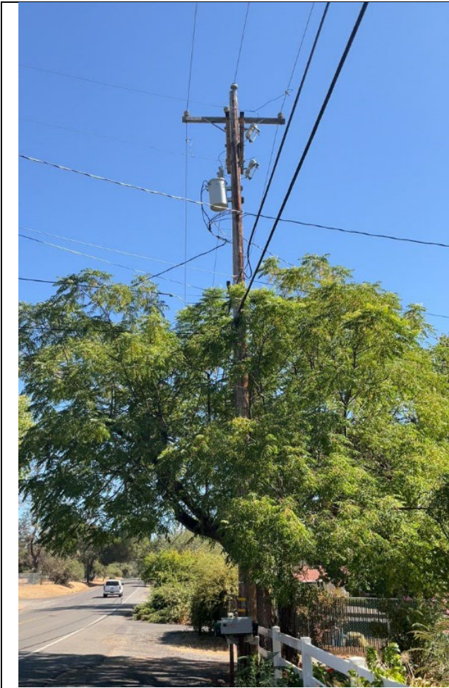
Item1IA1mg1: General photo of overall area.
