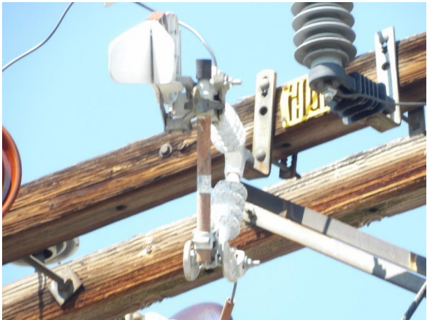
Item1IA1Img2: Expulsion Fuse Present
