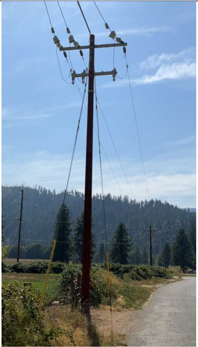
Item1IA1Img2: Overall Pole
