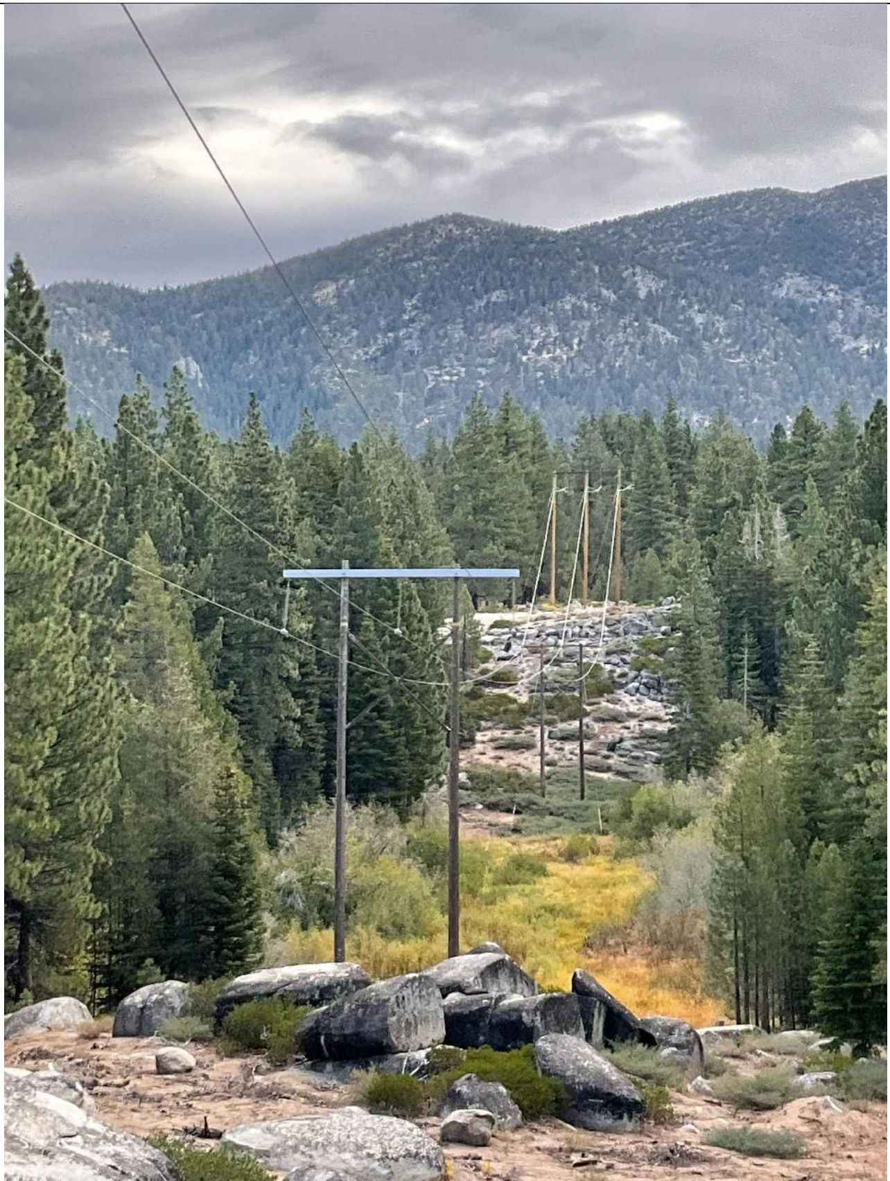
Item1IA1Img4: Overall section of 120 kV transmission line 111 with no distribution conductors
