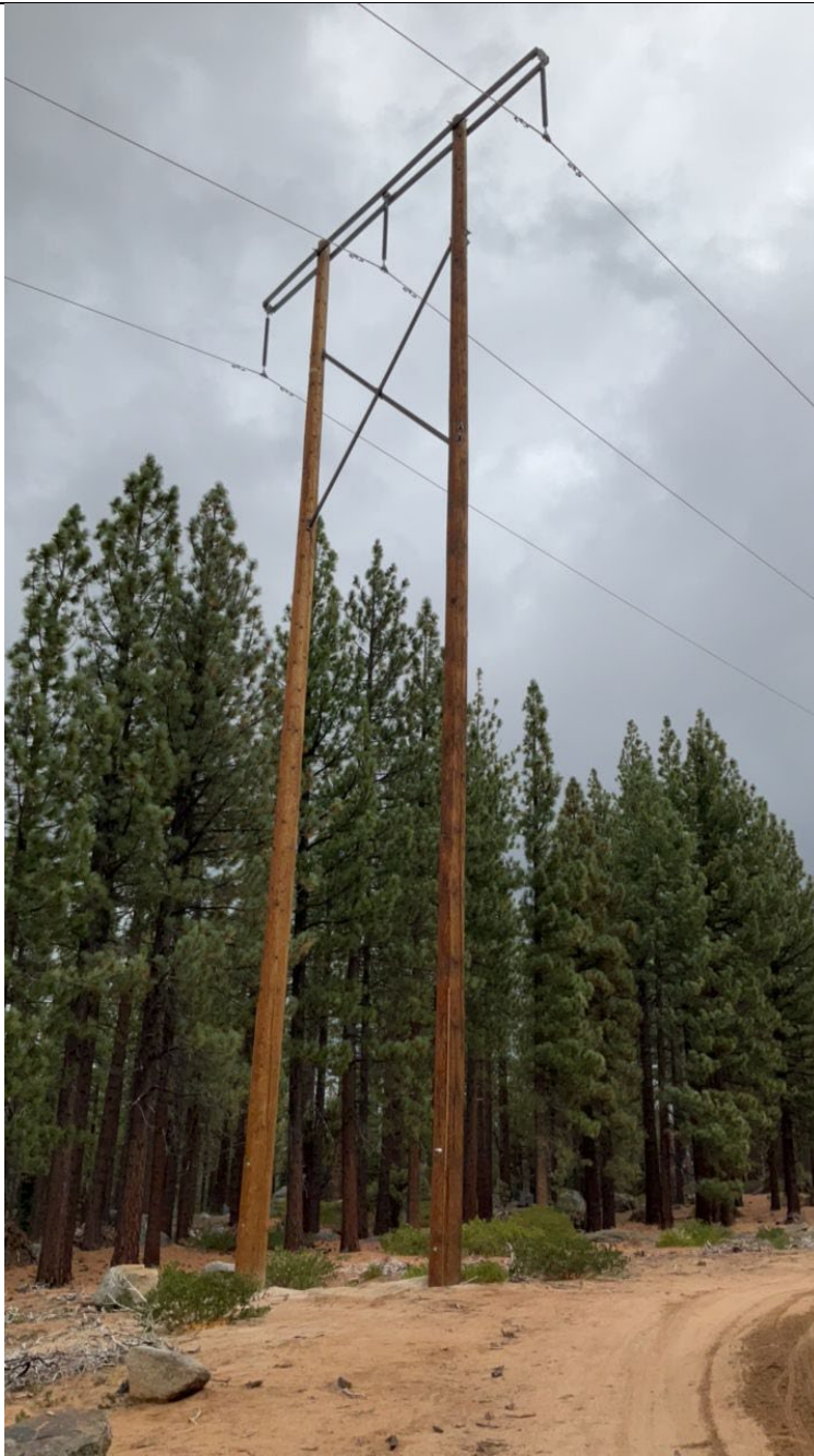
Item2IA1Img3: New steel crossarms for 120 kV transmission structure with no distribution conductors
