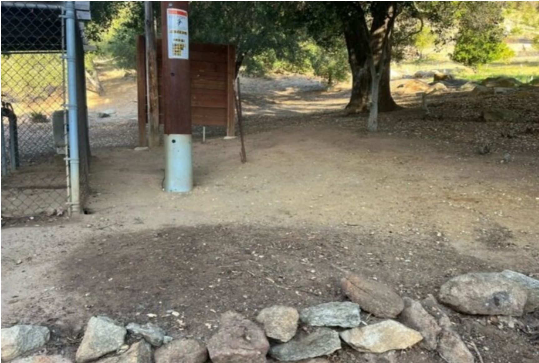
Figure 3: Image of post-pole clearing activity at Pole P814864 completed 11/25/24.
