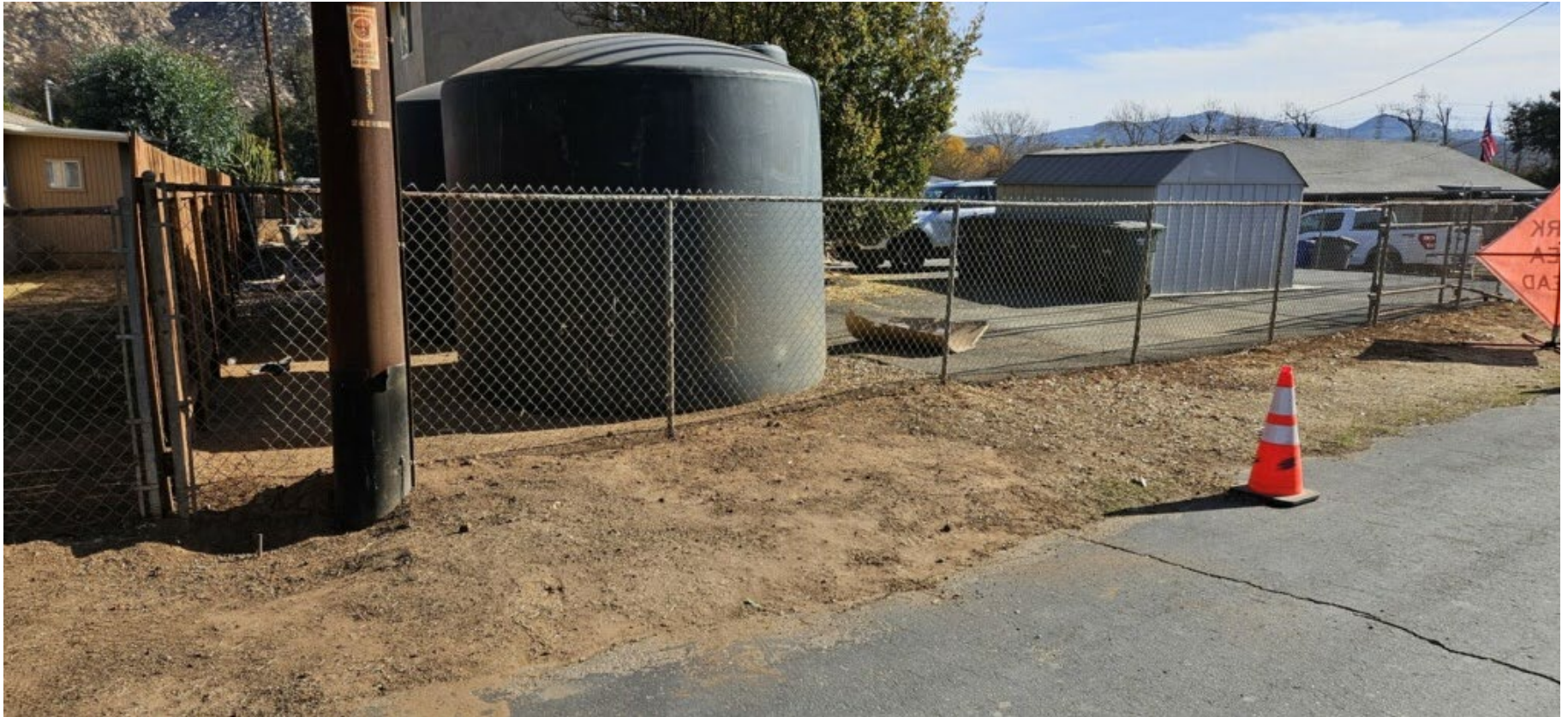
Figure 1 continued: SDG&E response post-NOV at P371207. Two photos showing re-clear work completed 12/16/24.
