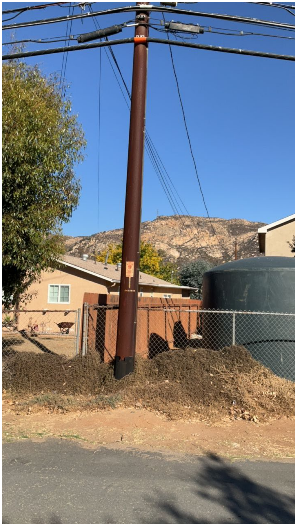
Item1Gimg2: Overall pole and vegetation surrounding the base of the pole.
