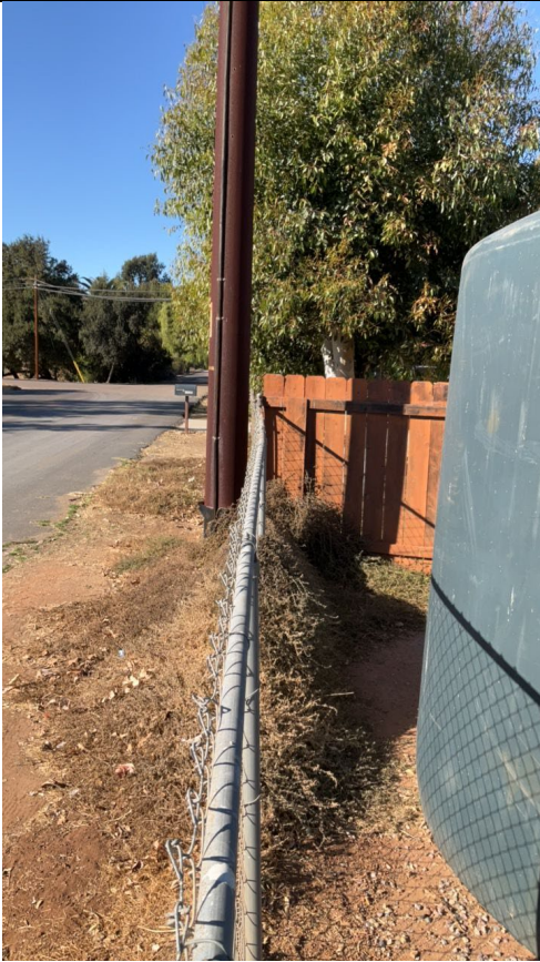
Item1GImg3: View of dying, flammable vegetation along fence within 10-foot radius of pole.
