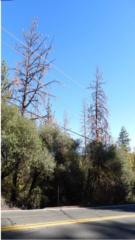
Item1IA1mg1: Photograph taken from across the street east from pole ID 121575549. The first tree is north of the conductors at 0.2 span and second, third, and fourth trees are north of the conductors at 0.4 span.
