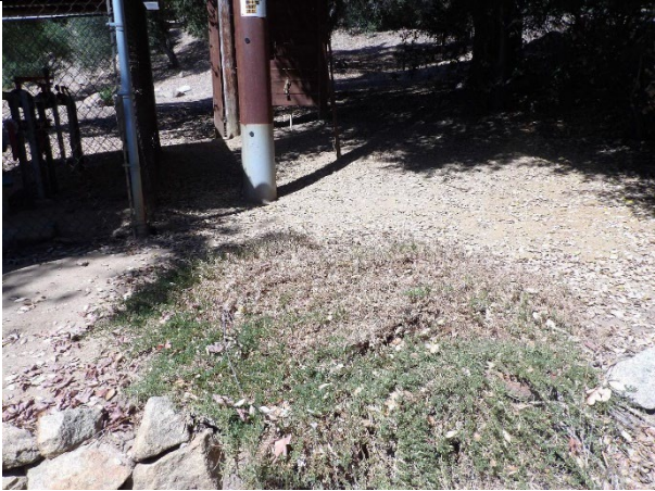
Item1GImg3: Vegetation within the 10-foot radius of the pole.
