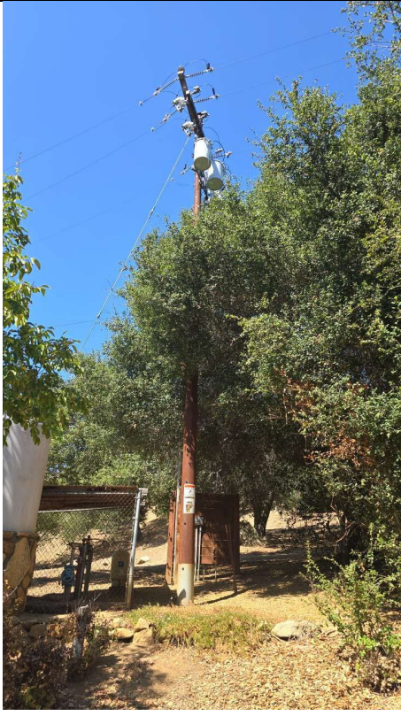
Item1GImg2: Overall pole and vegetation near the base of the pole.
