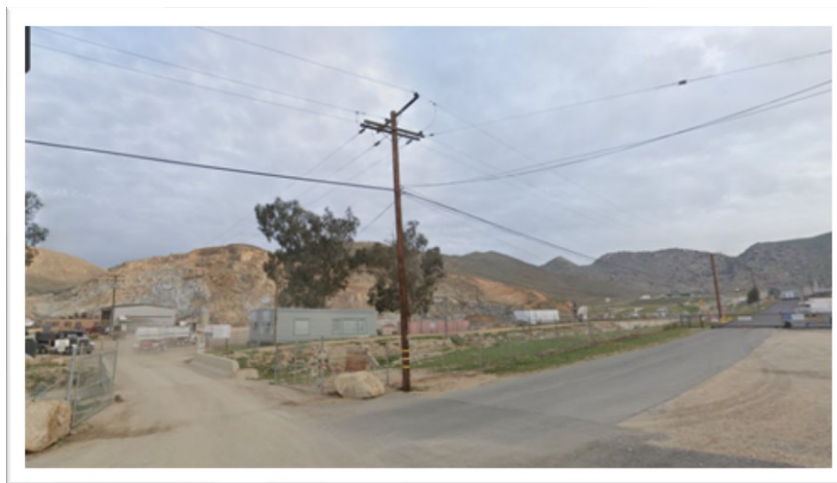
Figure SCE 6-17 - Photo of Location Confirms Need to Convert Designation from Severe Risk to High Consequence
