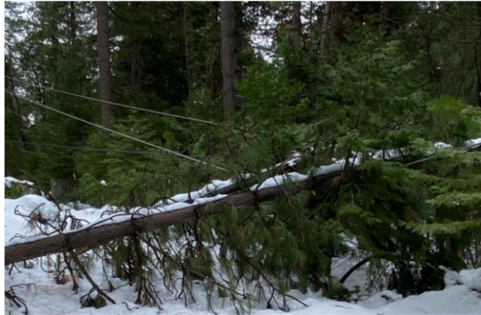
Figure CC-4 PG&E Covered Conductor Effectiveness – Example 3
