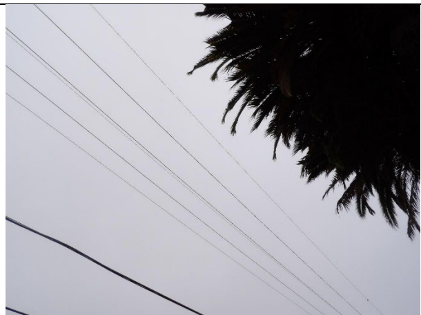
Item1IA1mg2: Photograph was taken looking up at horizontal distance. Photograph depicts a view of the two-foot distance between the palm and conductors.
