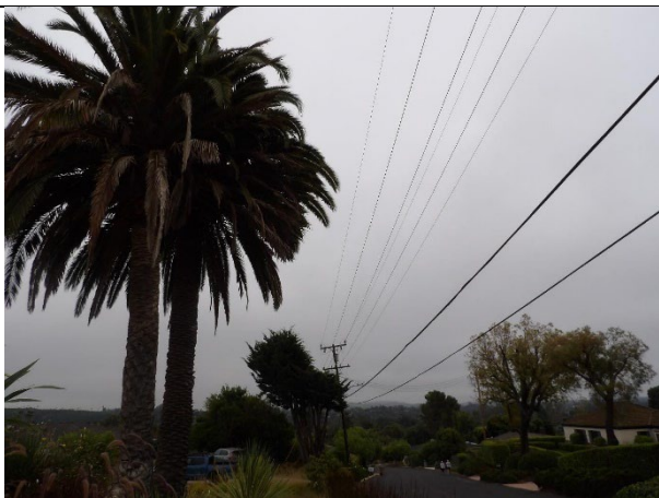
Item1IA1mg1: Photograph was taken facing southeast. Photograph depicts a view of the two-foot distance between the palm and conductors.
