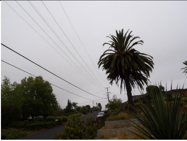
Item1IA1img3: Photograph was taken facing northwest. Photograph depicts a view of the two-foot distance between the palm and conductors.
