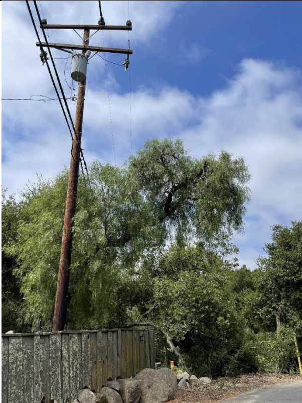
Item1IA1img2: Overall pole 205829E.
