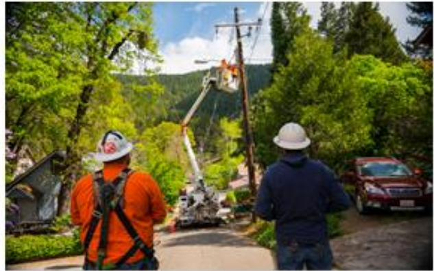
Figure 8-13: Line Crews at Work
