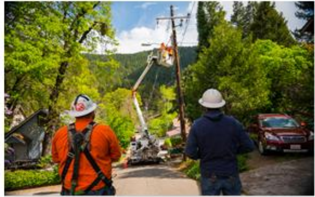
Figure 8-13: Line Crews at Work
