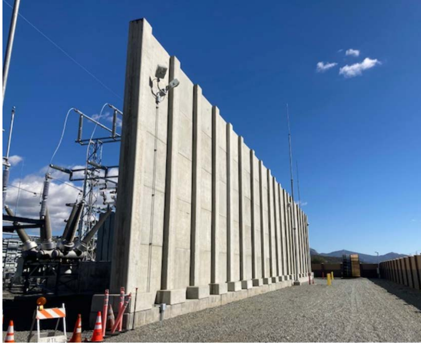
Figure HWT 8.1.2--1. Transformer Fire Barrier Wall
