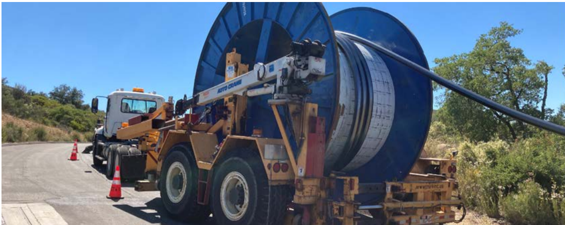
Figure HWT 8.1.2--2. Undergrounding of 0.02 mi overhead section of line
