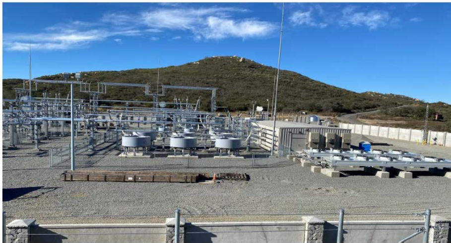
Figure HWT 8.1.2-4. Suncrest SVC hardscape and perimeter wall
