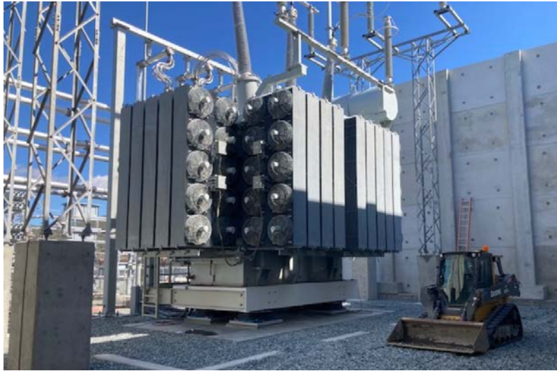
Figure HWT 8.1.2-3. Transformer Seismic Isolation Pad
