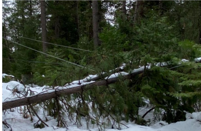
Figure F-4 PG&E Covered Conductor Effectiveness – Example 3
