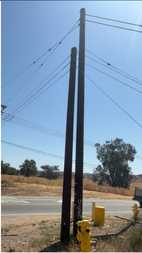
Item1IA1img1: No Covered Conductor Present
