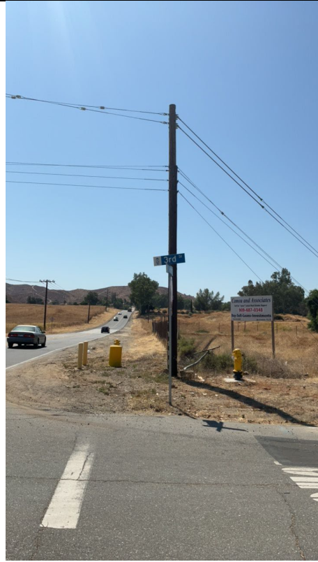
Item1IA1img2: No Covered Conductor Present
