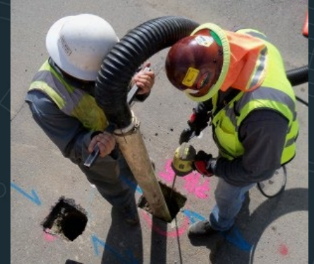
Vac-truck & Hand Excavation
