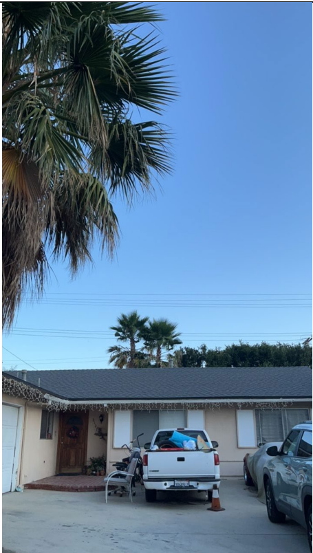
Item1IA1Img2: California palms breaking minimum clearance requirements. Photograph was taken from the south side of the sidewalk along Cheam Avenue facing 319.8 degrees northwest.
