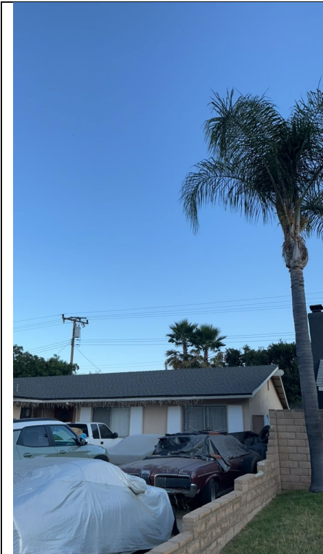
Item1IA1Img1: California palms breaking minimum clearance requirements. Photograph was taken from the north side of the sidewalk along Cheam Avenue facing 298.3 degrees northwest.
