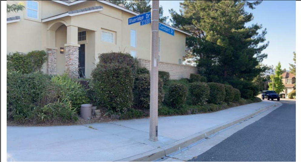
Item1Gimg1: Overall view of location showing a street light pole with no electrical equipment
