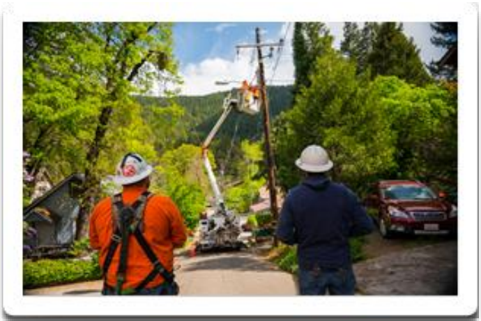
Figure 8-13 Line Crews at Work
