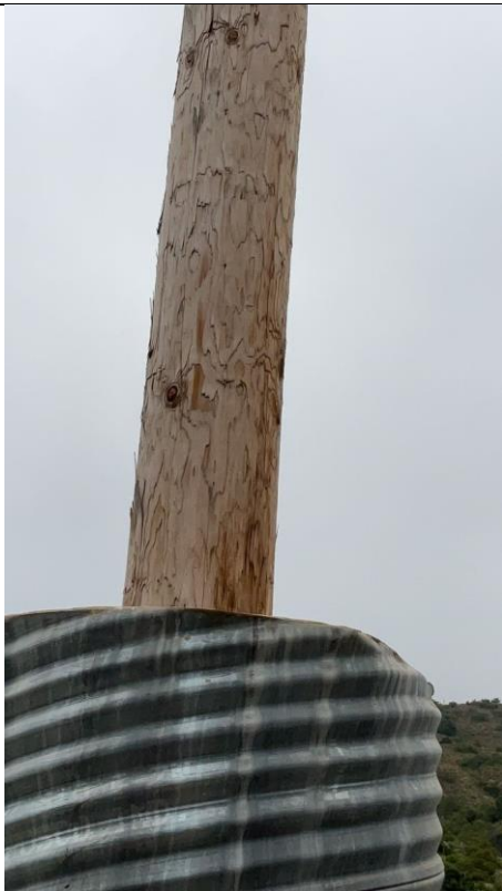
Item3GImg1: Missing Pole ID
