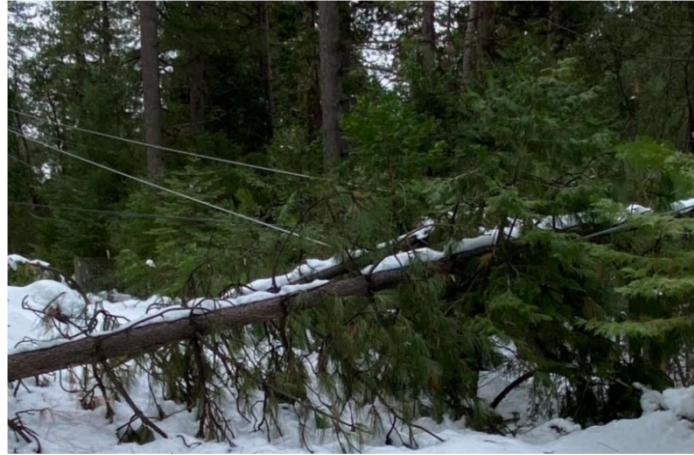
Figure F-4 PG&E Covered Conductor Effectiveness – Example 3
