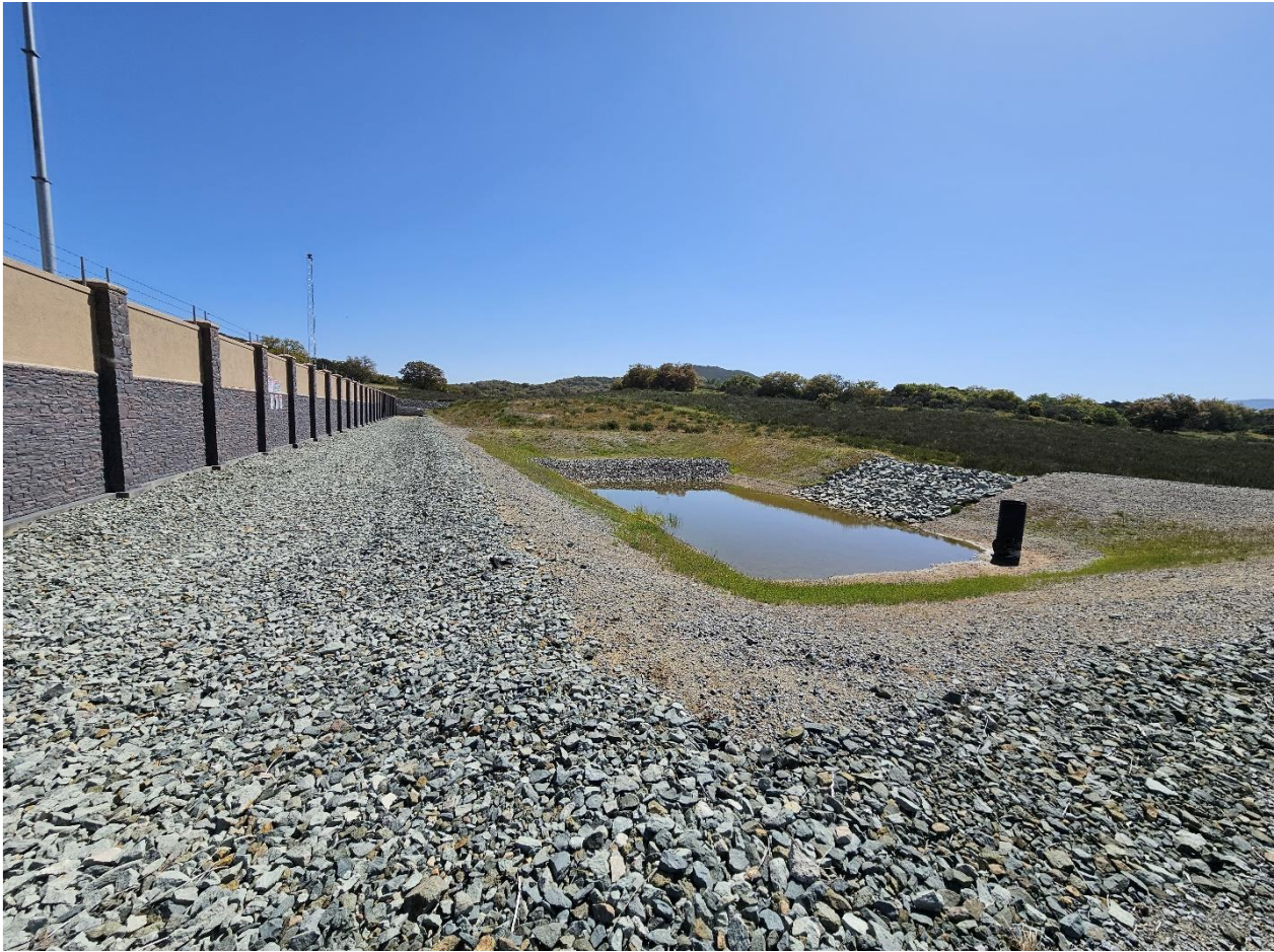
View of retention pond and firebreak facing NE
