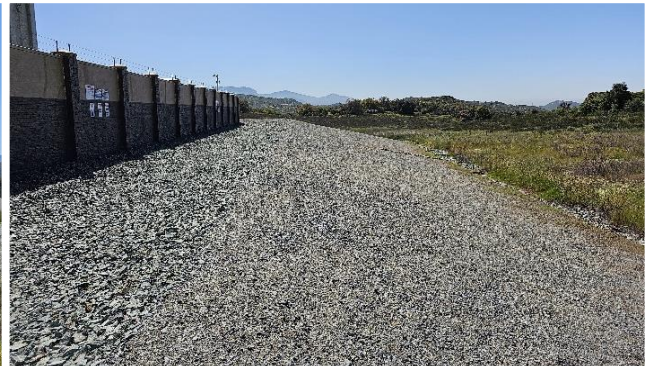
Firebreak outside SW Wall
