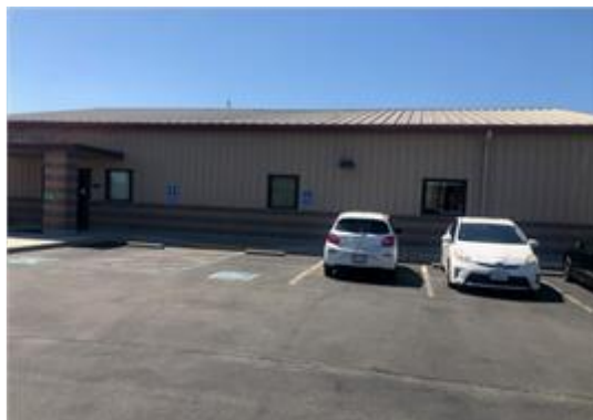
Figure 19 – Office and Administration Building
