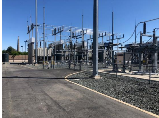
Figure 26 - 230/180 kV Transformers
