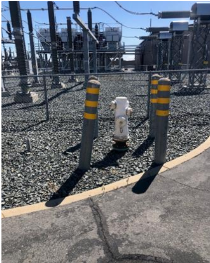
Figure 27 - Fire Hydrant w Vehicle Impact Protection
