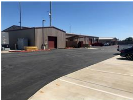
Figure 22 - Spare Parts, Converter Hall, and Control Center
