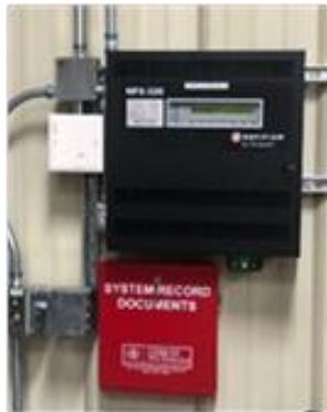
Figure 11 – Control Panel for suppression system
