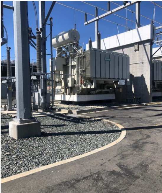
Figure 29- 230/180 kV Transformer
