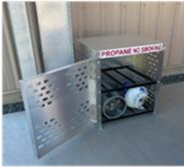
Figure 8 – Compressed gas storage
