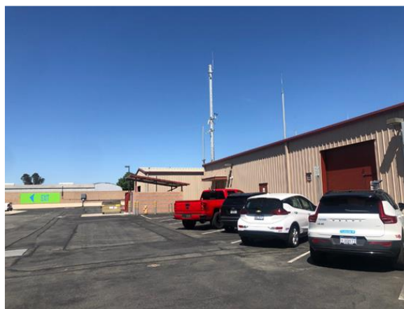
Figure 17 – Converter Hall, Spare Parts Building & Weather Station
