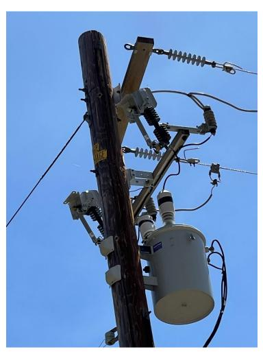
**Liberty Response 2 -** As stated in its initial response to Energy Safety NOV\_LU\_CAC9\_20221019\_1218, Liberty has replaced the expulsion fuse on pole ID 269462 with a non-expulsion fuse alternative to reduce wildfire risk. The following photo shows the completed work at this location:
