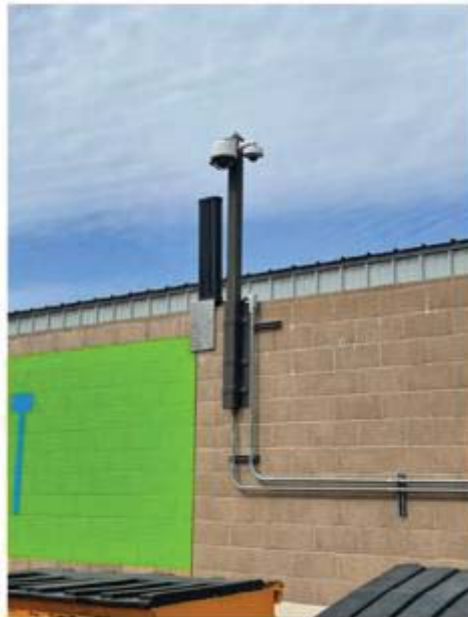
Figure TBC 8.1.2- 1. Perimeter Wall and Cameras
