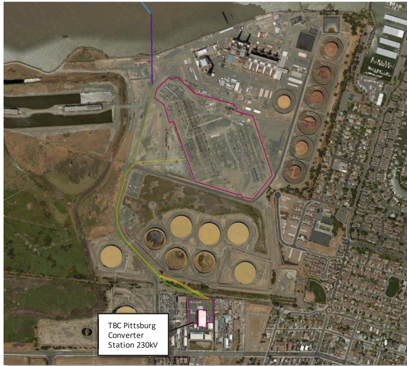
Figure TBC 5.1- 5. Overhead View of TBC Pittsburg Station
