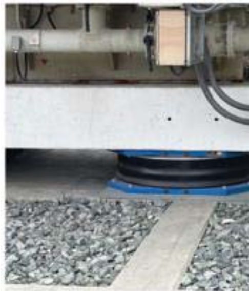
Figure TBC 8.1.2- 6. Close up of Isolator
