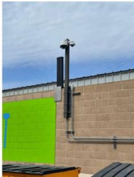
Figure TBC 8.1.2- 1. Perimeter Wall and Cameras
