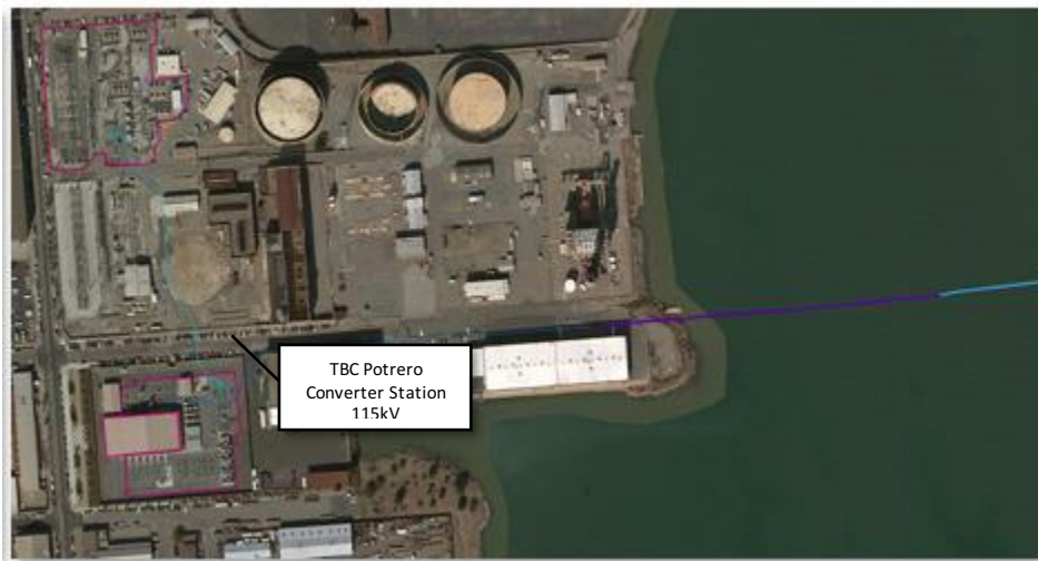
Figure TBC 5.1- 3. Overhead View of TBC Potrero Station
