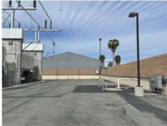
Figure TBC 8.1.2- 3. Hardscaped AC yard
