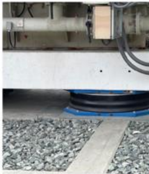
Figure TBC 8.1.2- 6. Close up of Isolator
