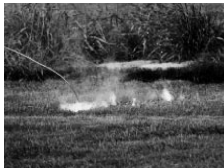
Figure 3 A downed conductor arcs to ground at Texas A&M University's Downed Conductor Test Facility
