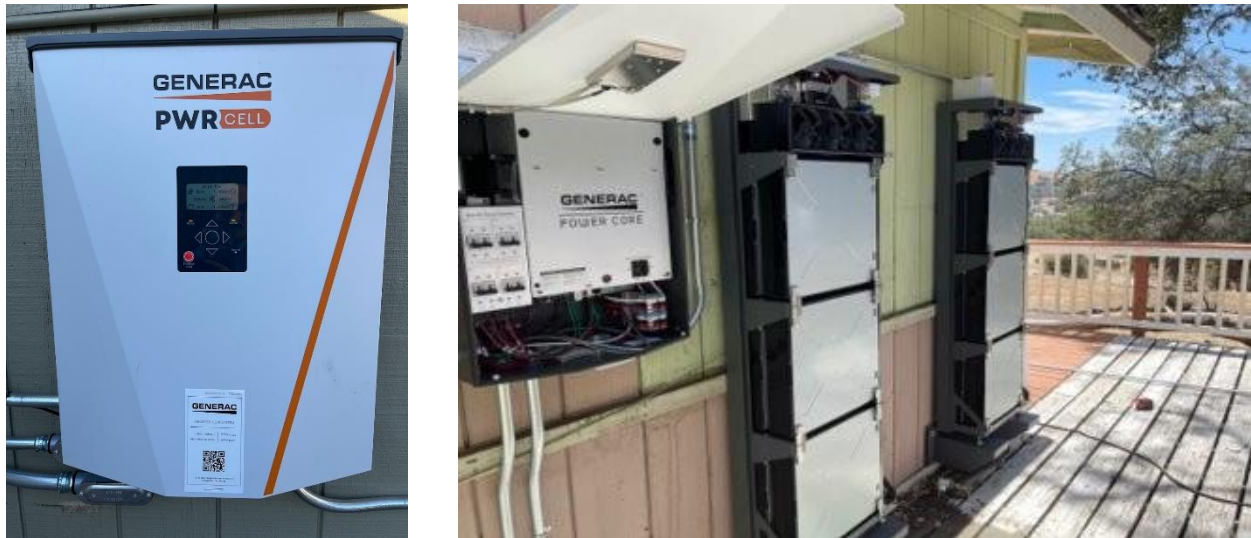
Figure 8-7: FPB Installation at Mobile Home Park Community
