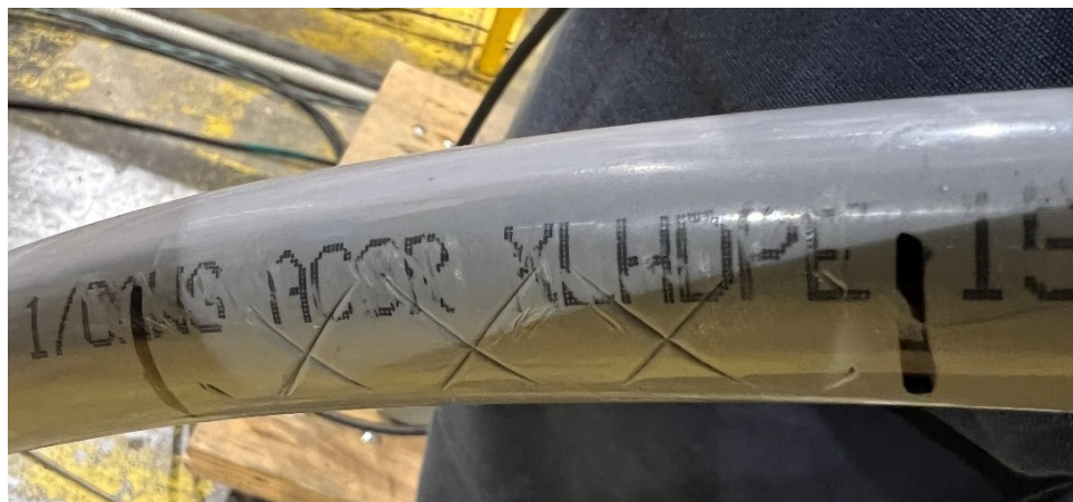
Figure 6-15: Sample 3.2.2 - 35 kV, 1/0 AWG ACSR Condition after Test
