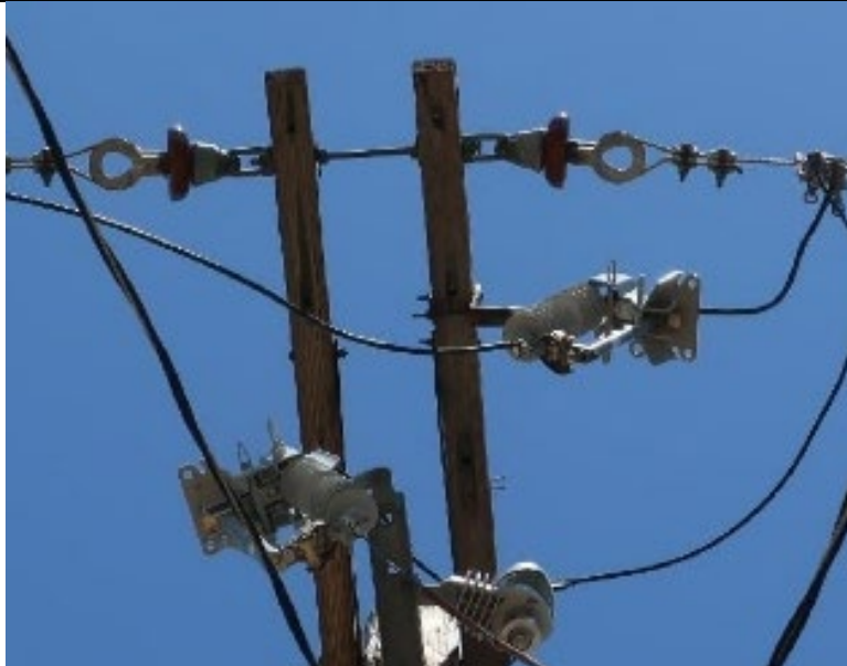
Item7IA1Img1: Overall view of one expulsion fuse and one Cal-Fire exempt fuse
