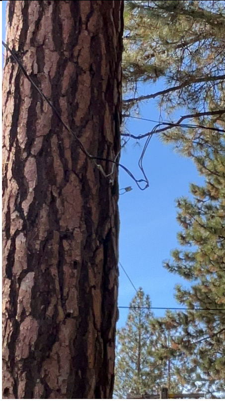
Item8GImg3: Close-up view of tree attachment.
