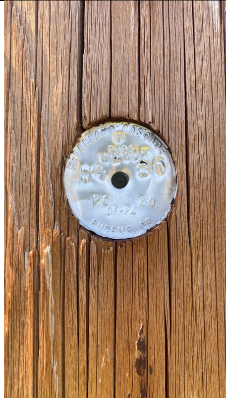
Item13IA1img4: View of pole brand showing a manufacture date of September 2006.
