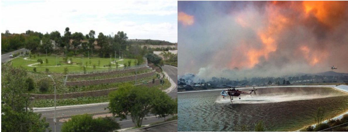
Figure 2: (a) Park Substation (b) Walnut Canyon Reservoir during Canyon Fire 2
