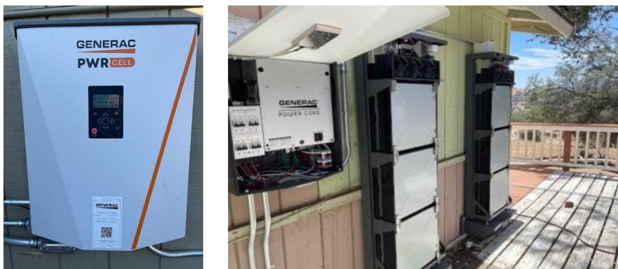
Figure 8-6: FPB Installation at Mobile Home Park Community
