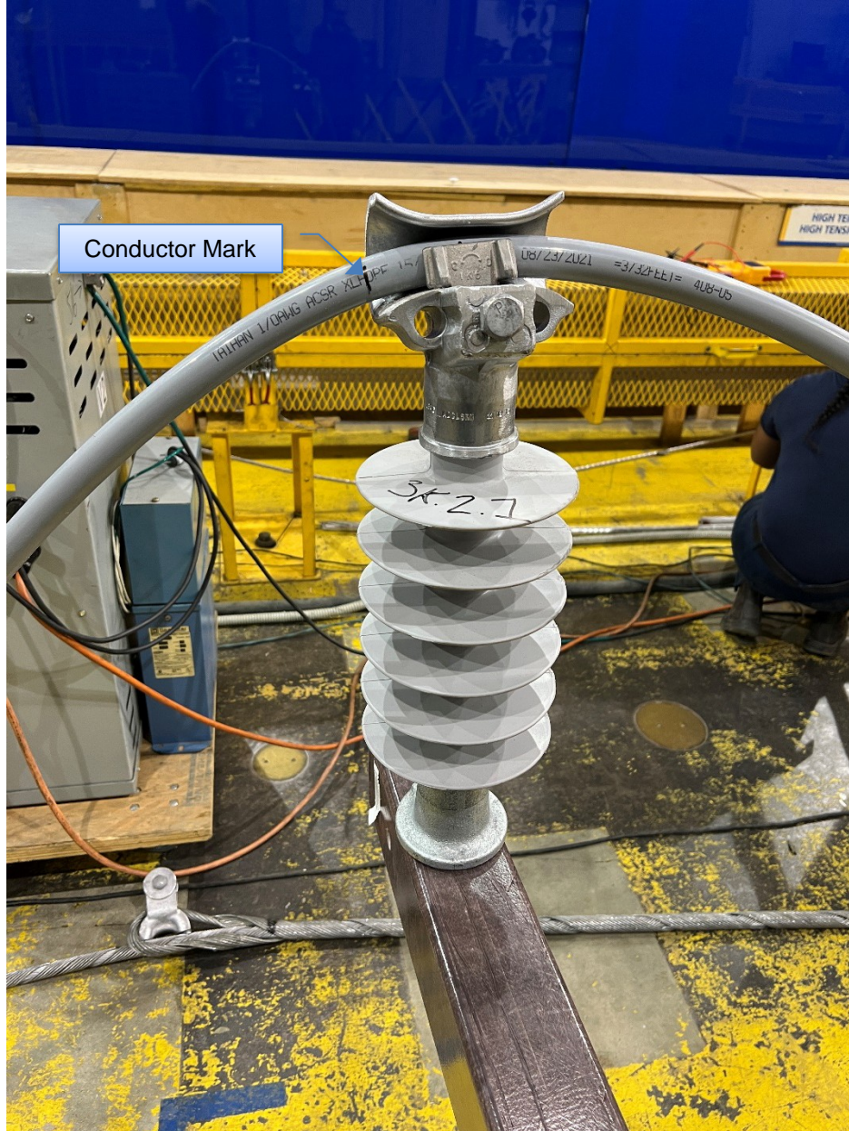
Figure 6-31: Sample 3K.2.1 – Insulator and Cross-arm Condition after Test
