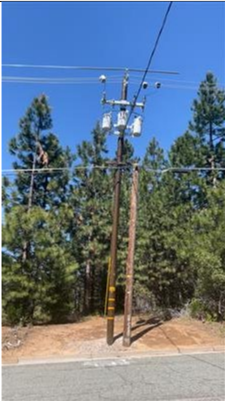
Item8GImg2: Overall Pole
