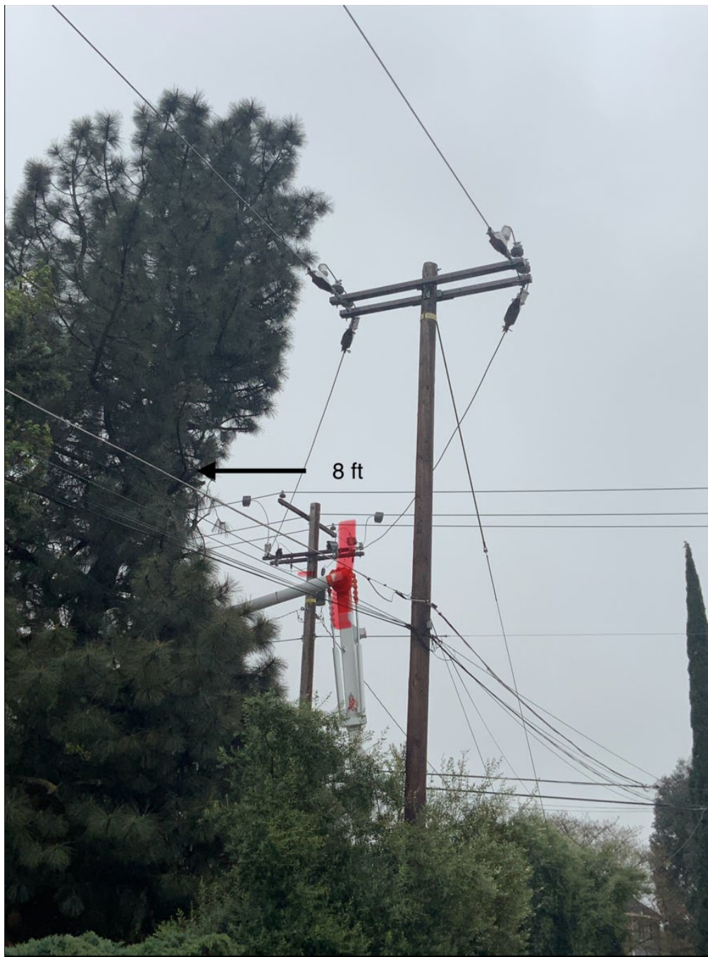
Post trim clearance established at 8 ft
