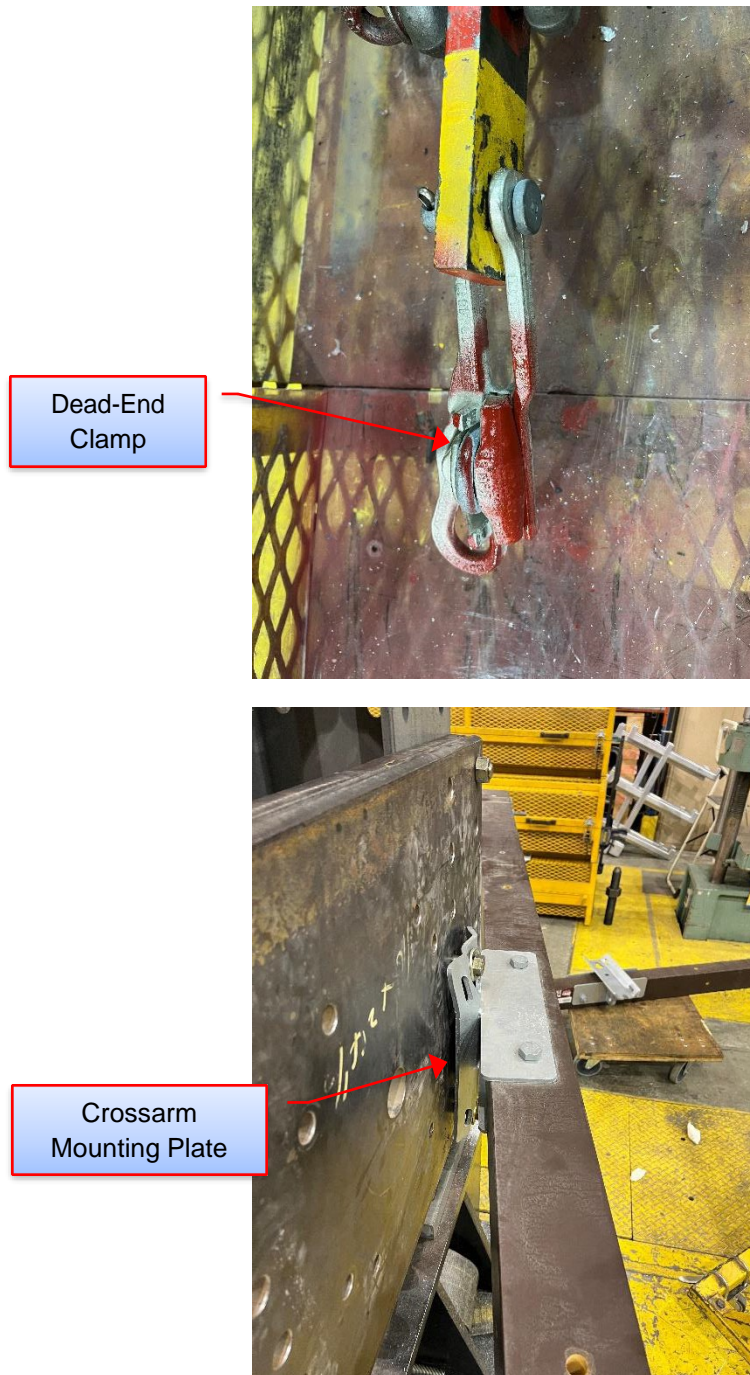
Figure 6-15: Sample 3.2 – Failure Location
