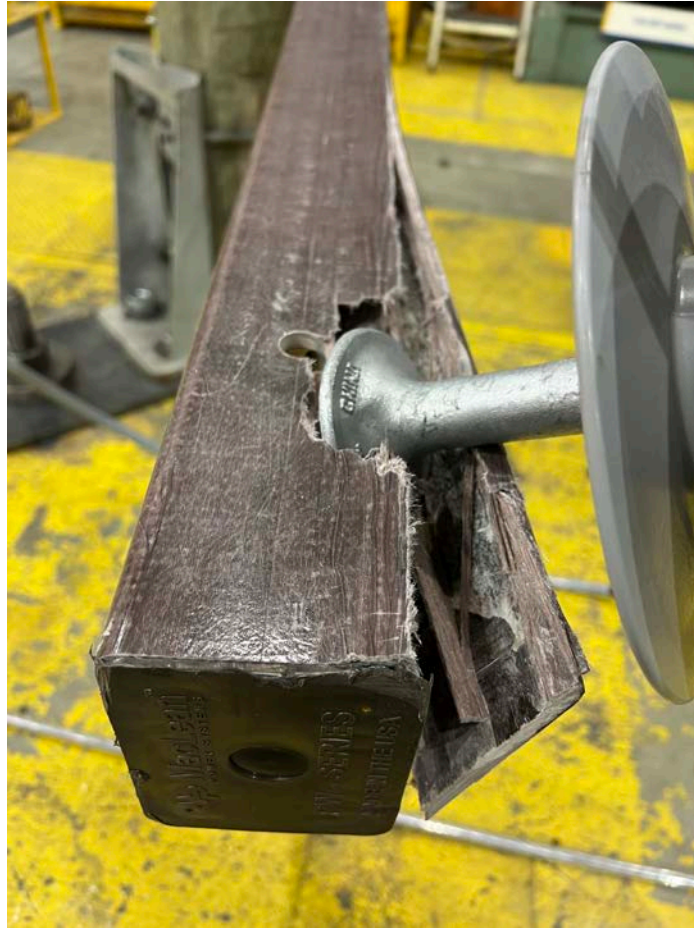
Figure 71. A representative post-test image showing pull-out of the insulator pin at final failure (17-kV 1/0 ACSR).
