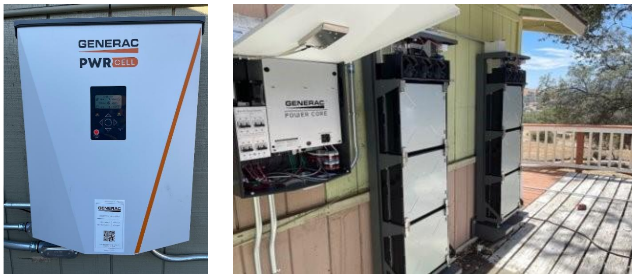
Figure 8-6: FPB Installation at Mobile Home Park Community
