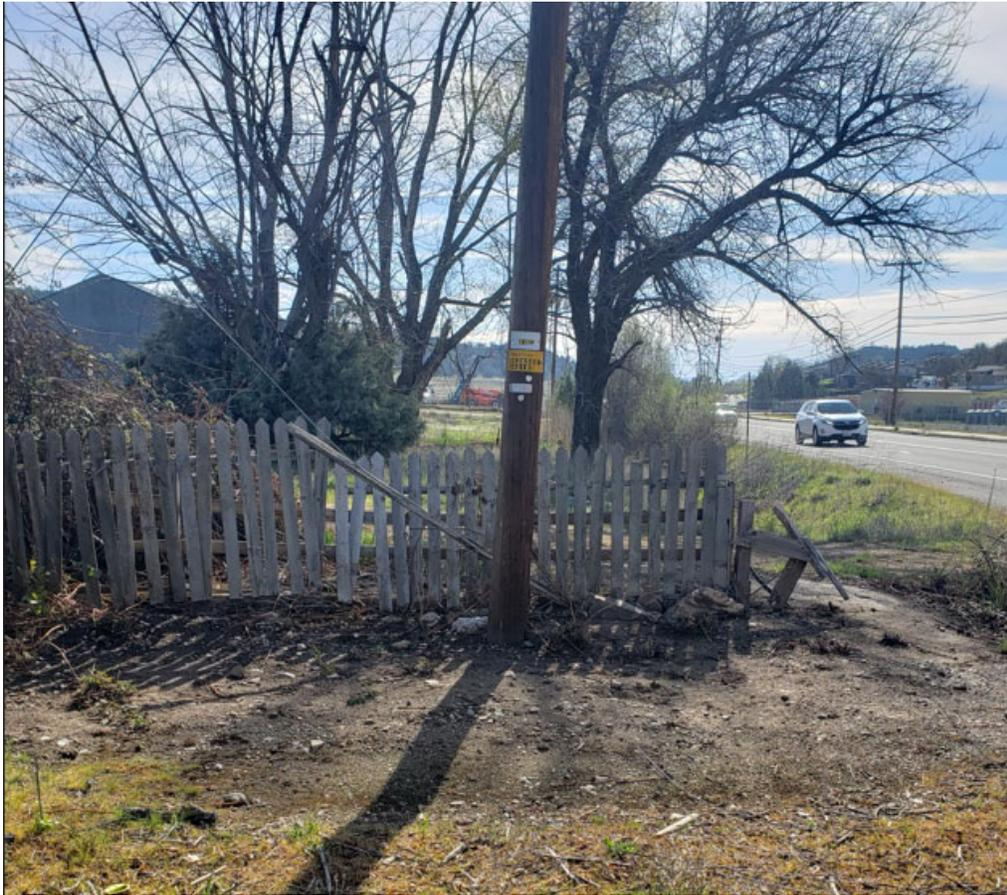
**Violation 2.** Energy Safety observed that in implementing WMP initiative number 8.2.3.1.2 – Pole Clearing, PacifiCorp failed to adhere to a required protocol of pole clearing to achieve required clearance at pole ID 06245007263000 at coordinates 41.71374976, -122.62534223. Energy Safety considers this violation for failure to adhere to protocol to be in the Minor risk category.
