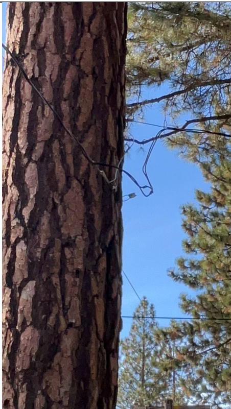
Item8GImg3: Close-up view of tree attachment.
