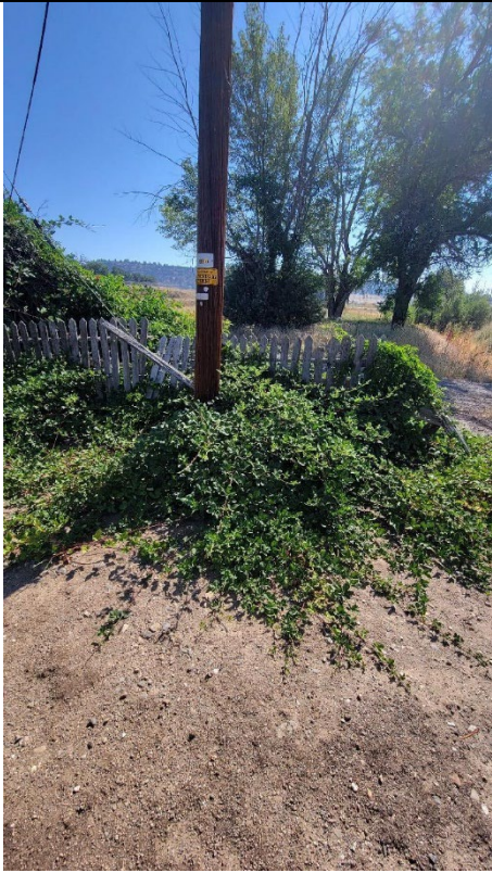
Item1IA1mg1: View of vegetation growing within a 10-foot radius of the pole.
