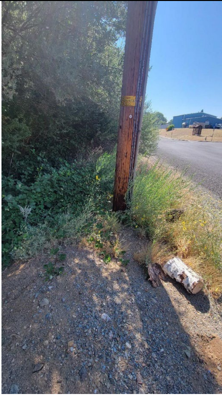
Item2IA1Img1: View of vegetation growing within a 10-foot radius of the pole.
