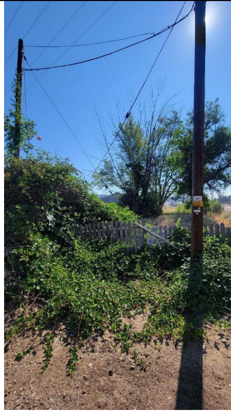
Item1IA1mg2: View of vegetation growing within a 10-foot radius of the pole.
