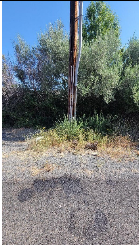
Item2IA1Img2: View of vegetation growing within a 10-foot radius of the pole.
