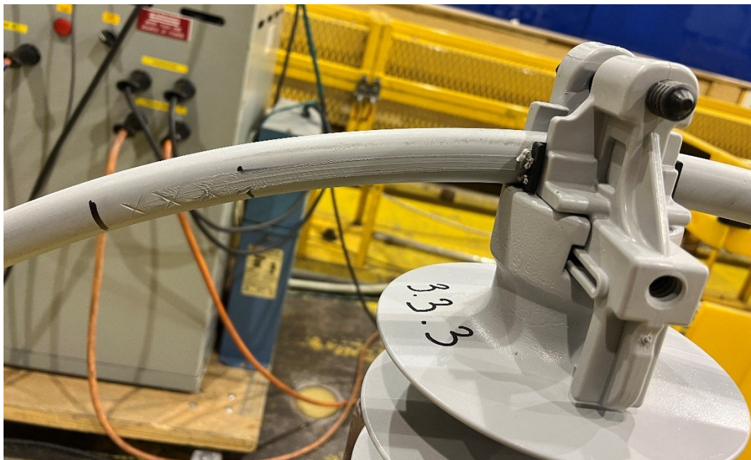
Figure 6-20: Sample 3.3.3 - 22 kV, 397.5 kcmil AAC Condition after Test
