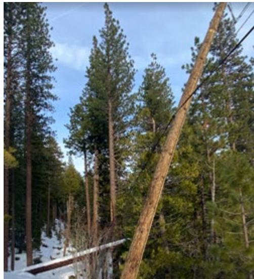
Upon finding the damage, the poles were reset to vertical and the damaged support brackets were replaced. No damage was found related to the conductor.
